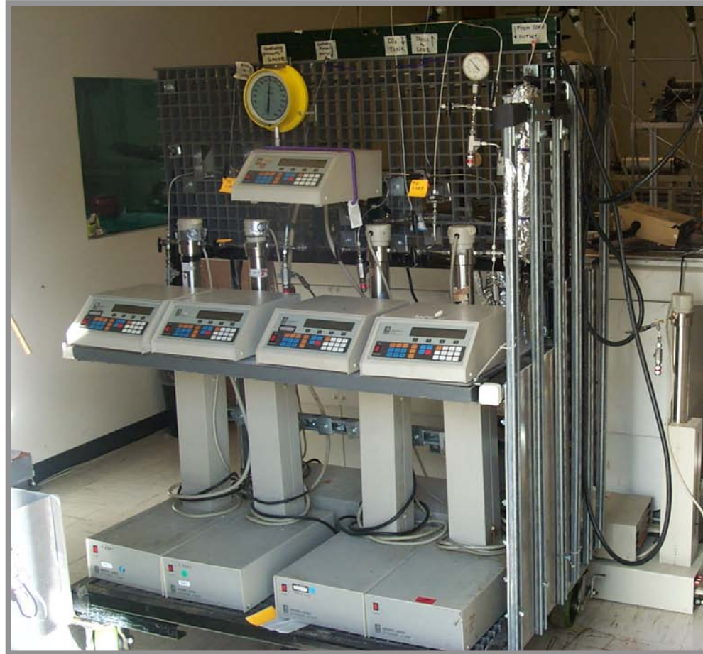
High Pressure Pumps
